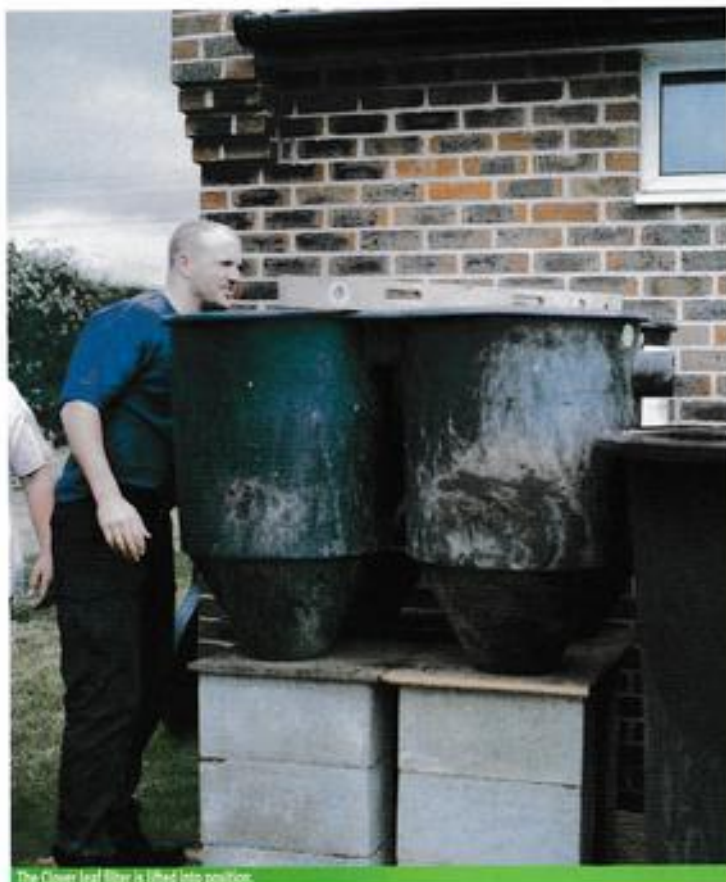
The Cover leaf filter is lifted into position.
